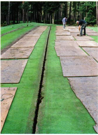
with the aim being to increase the removal of water from the subsoil to allow the topsoil to drain at its optimum rate.
